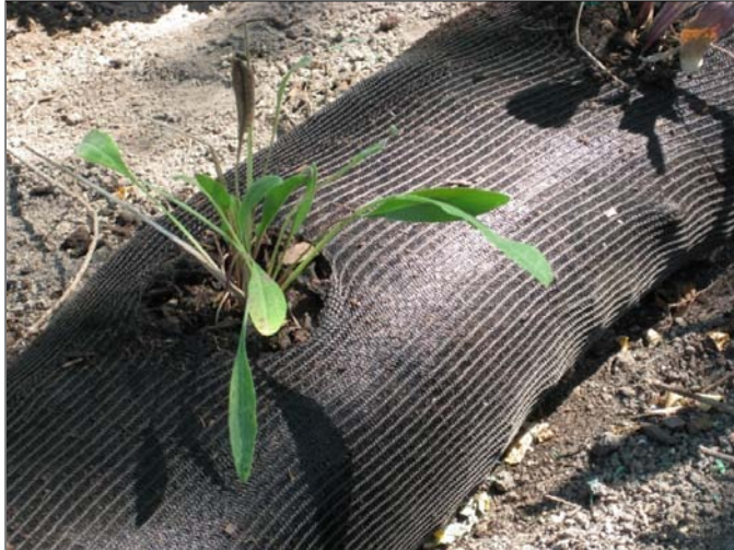
Example of Filtrexx® soxx planted and filled with compost.
