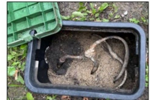
Existing Pull Box
