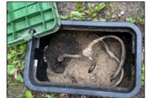
Existing Pull Box
