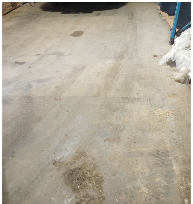
Figure 20 Typical Interior Concrete Slab in Main East-West Portion of the Building
