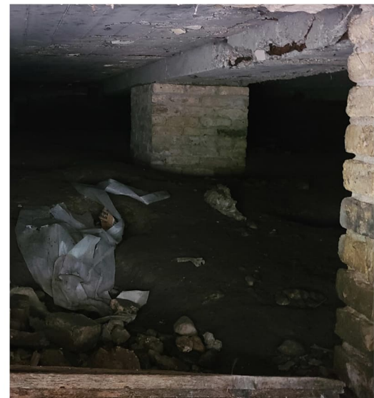
Figure 11 Typical Brick Interior Slab Support Pier
