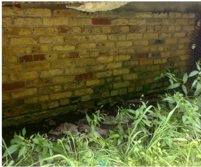
Figure 10 Typical Brick Perimeter Foundation Wall
