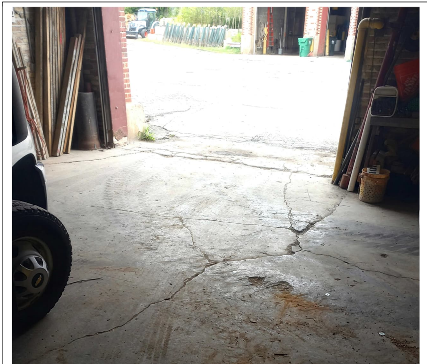
Figure 21 Interior Concrete Slab at Northeast
