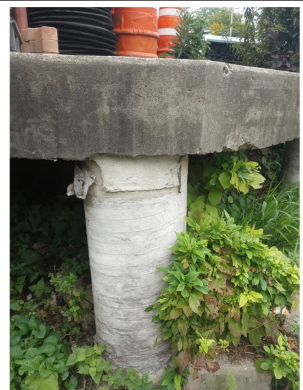
Figure 13 Current Circular Concrete Piers at West Shipping Platform
