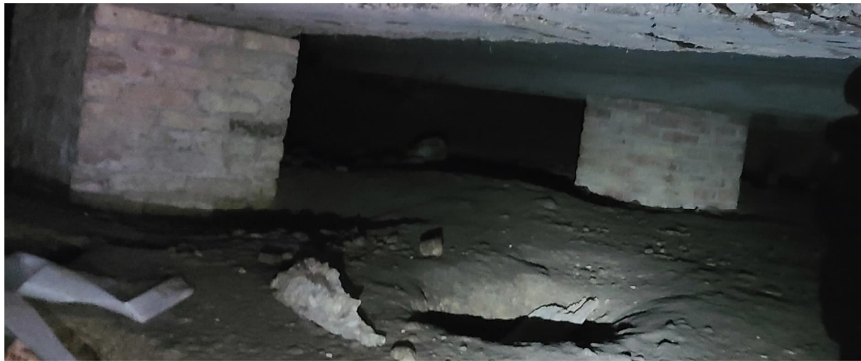
Figure 34 Brick Pier Foundations Below Interior Building Slab
