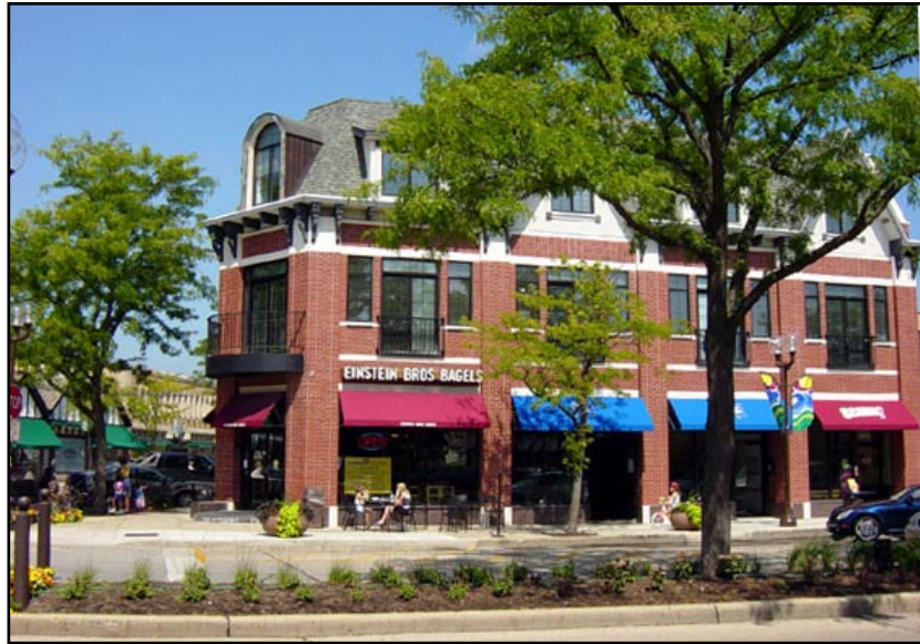
Corner building with attractive details such as decorated cornices, cast-iron balcony railings, dormers, and signs incorporated into sign bands.
