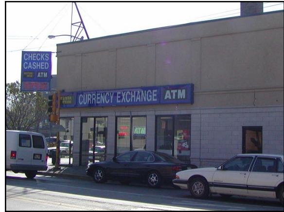
Large blade sign with excessive support structure.
