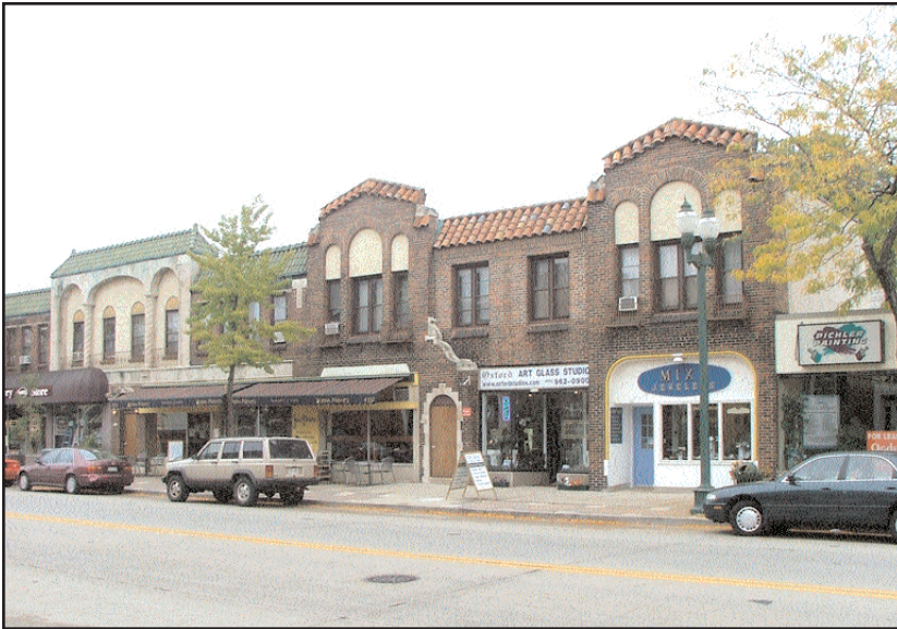
A commercial strip along North Oakland with first-floor restaurants and shops and residential units above.
