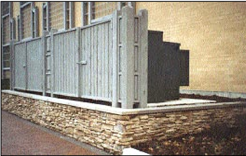
Screened utility area.
