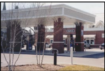
Gas station design shall incorporate quality materials and locate pumps in the rear when feasible.
