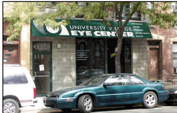
Cinder/concrete block as main building material is not allowed. Decorative block may be used for limited accent and trim.
