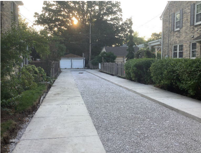
Alley 3 Finished Concrete and Stone Base
