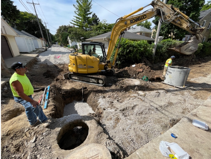
Alley 3 Storm Sewer
