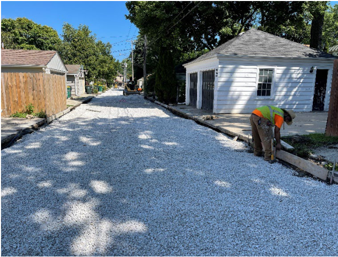
Alley 3 Concrete Grading
