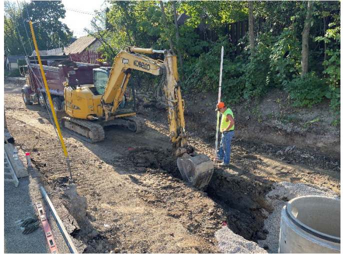
Alley 6 Storm Sewer
