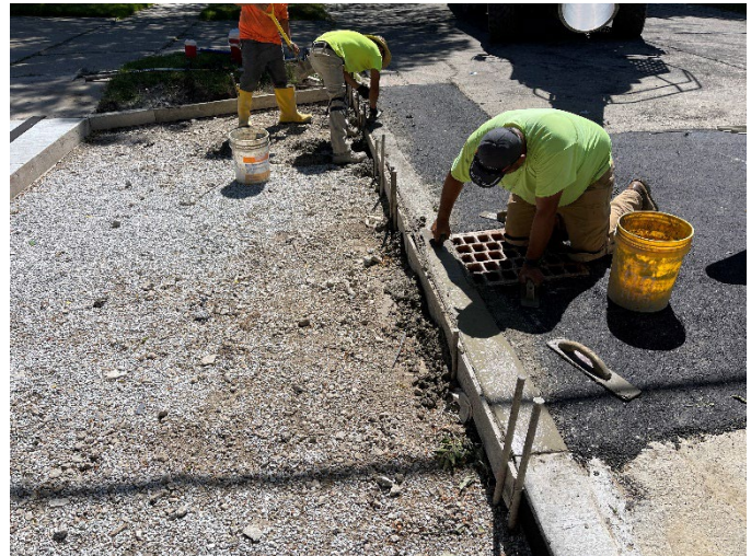
Alley 2 Concrete Curb and Gutter
