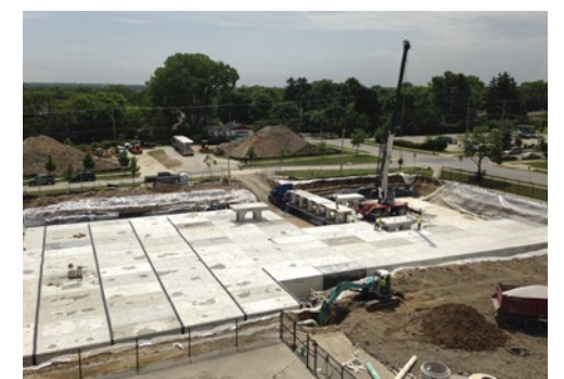
Westlawn Garden Project To Install Underground Detention
